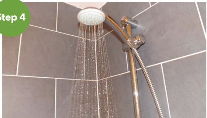
Reattach the showerhead and hose then run the water for a few minutes to get rid of the disinfectant. You are then good to go!
