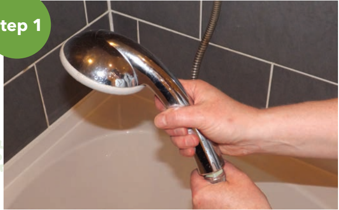
Disconnect the showerhead.
