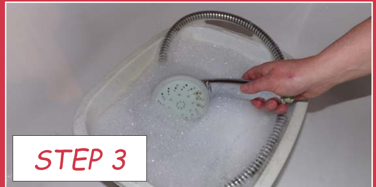
Steep the showerhead and the hose in a basin of warm water and disinfectant for about 15 minutes.
