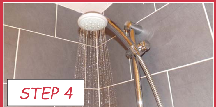
Reattach the showerhead and hose then run the water for a few minutes to get rid of the disinfectant. You are then good to go!
