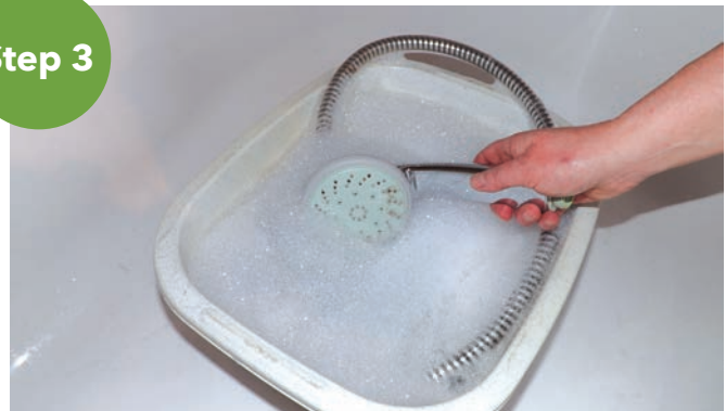
Steep the showerhead and the hose in a basin of warm water and disinfectant for about 15 minutes.
