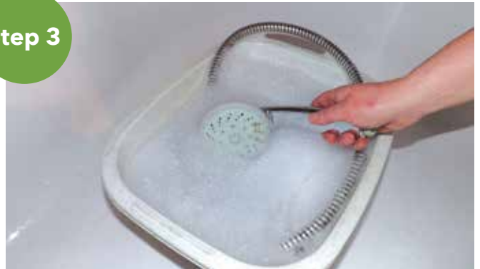
Steep the showerhead and the hose in a basin of warm water and disinfectant for about 15 minutes.
